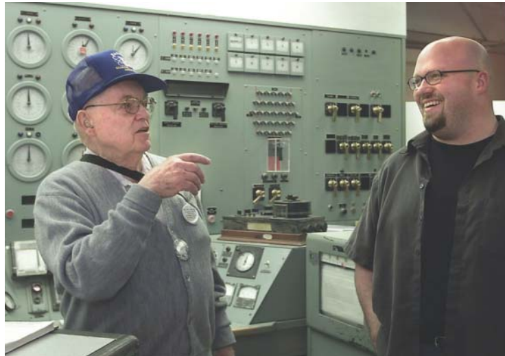
Retired B Reactor instrument supervisor, Dee McCullough, tells a visitor how the control panel worked.
